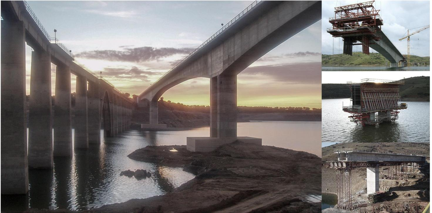
The existing Manzanal del Barco Bridge was built in 1935 to replace an older 1927 bridge which had been submerged in the reservoir after the construction of the Ricobayo Dam. The bridge has a 50.0m span central arch, and eight 25.0m approach spans from each shore. The 3.40m deck width causes traffic problems and widening proposals were initially rejected in a preliminary stage.
